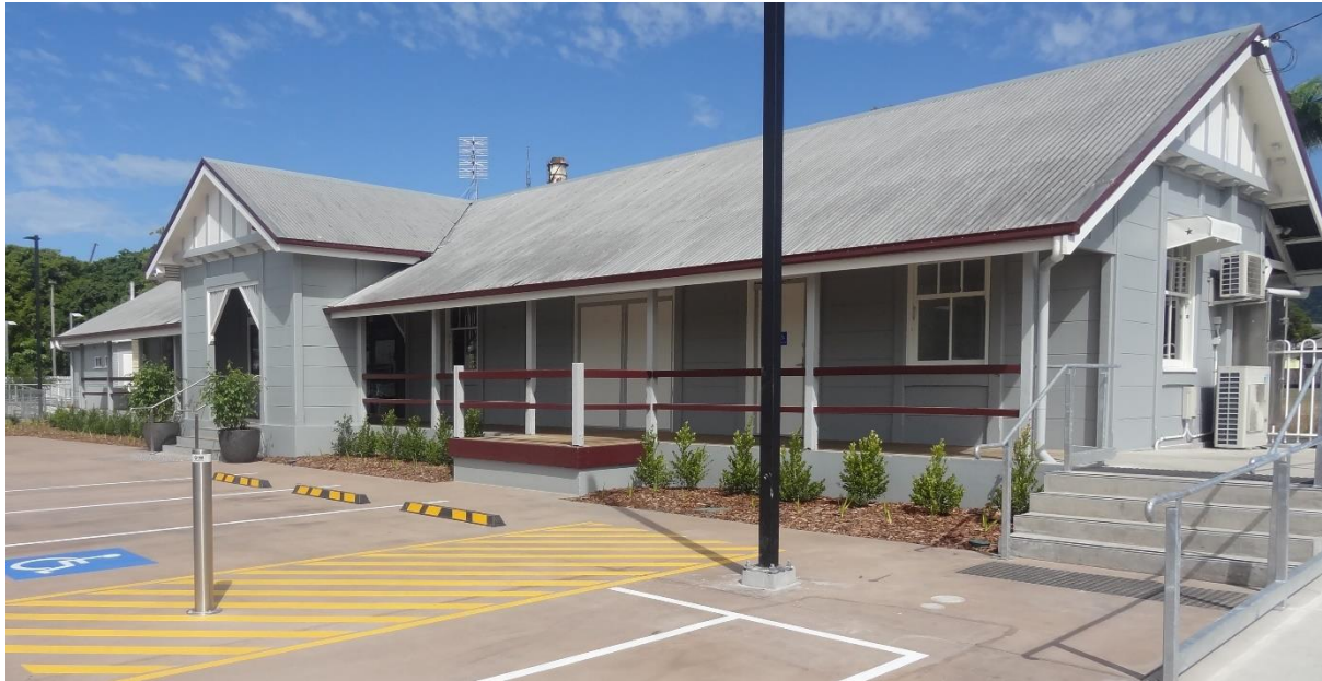
A view of the new Mackay District Visitor Information Centre which will open for business on July 1. The centre is in the old Sarina Railway Station, which has been refurbished as part of the redevelopment of the Field of Dreams parkland over the past 12 months.
